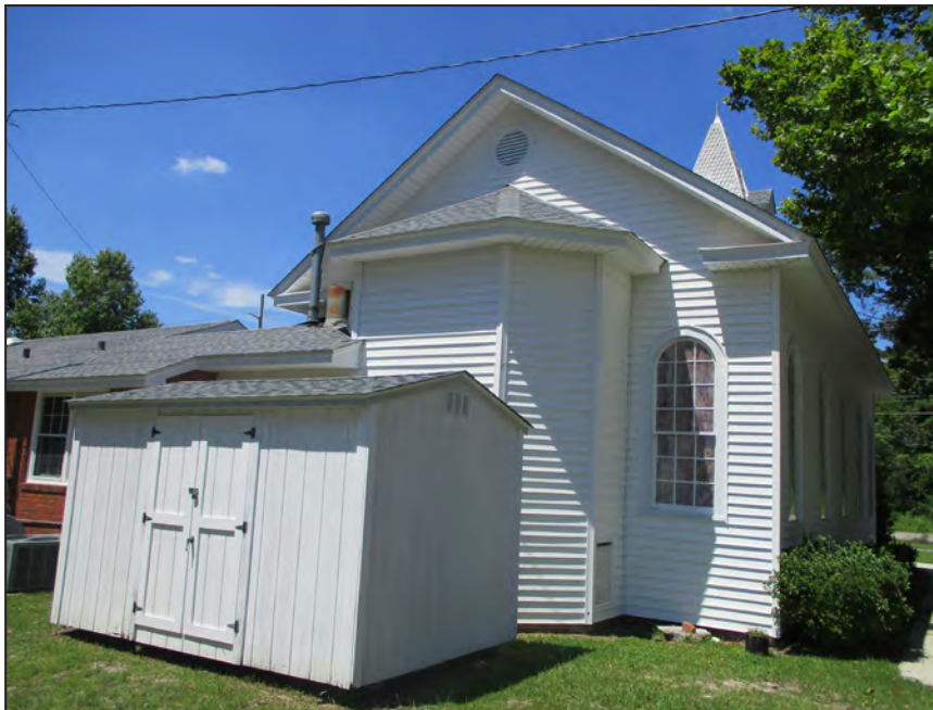
Photograph 5: Rear (southwest) elevation of Concord United Methodist Church looking north. (2018)
