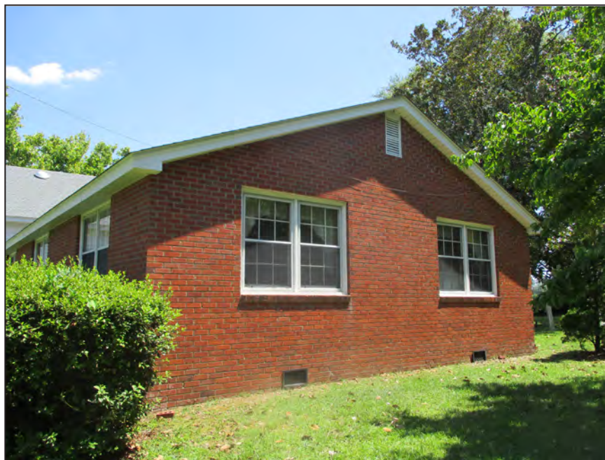
Photograph 11: Ca. 1959 addition northwest elevation. (2018)
