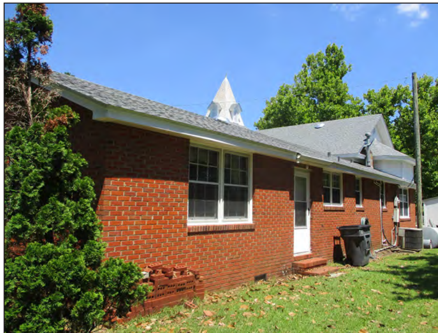
Photograph 12: View of ca. 1959 addition's southeast (rear) elevation; looking east. (2018)
