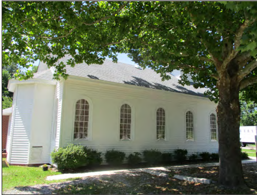
Photograph 6: Southeast elevation of Concord United Methodist Church looking northwest. (2018)
