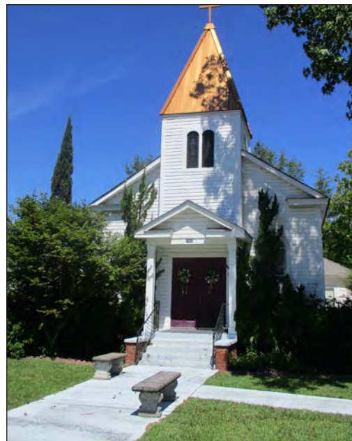
Photograph 17: Bethel United Methodist Church. (2018)
