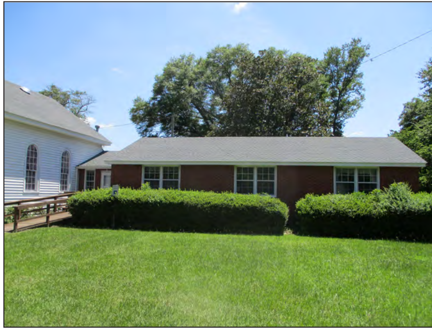
Photograph 10: Ca. 1959 addition northeast elevation. (2018)
