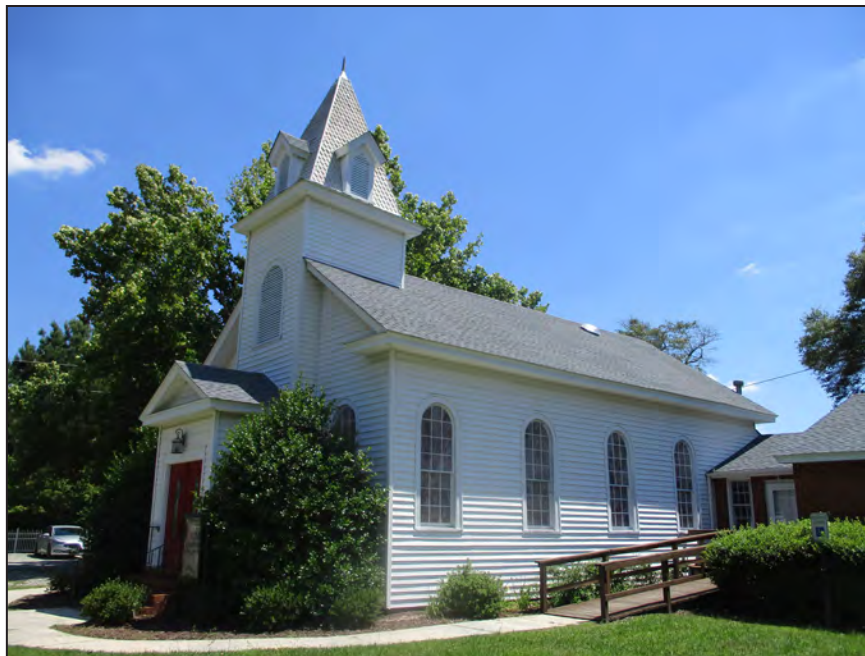
Photograph 7: Northwest elevation of Concord United Methodist Church looking south. (2018)
